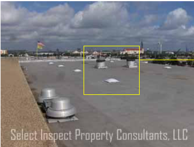
↑ most of the main warehouse roof was satisfactory
