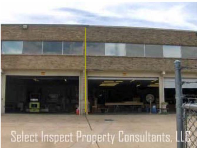
↑ structural addition implied by variant tone of brick & roofline & driveway control-joint
