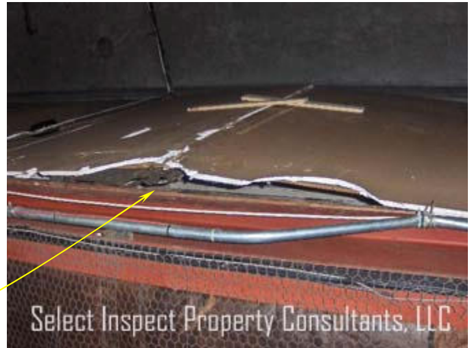
↑ unsteady/hinged wall viewed from below
