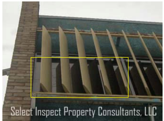
↑ cracked window discovered at the office
